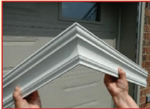
**Create perfectly fitting exterior crown molding joints**
