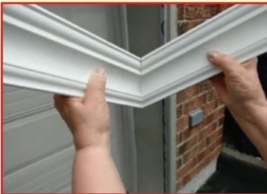
**Create perfectly fitting interior crown molding joints**
