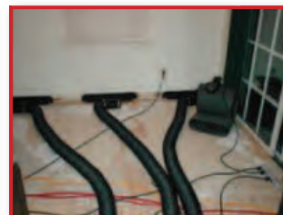
Monitor water damage restoration
