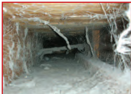
Inspection of hard-to-reach and hard-to-see areas
