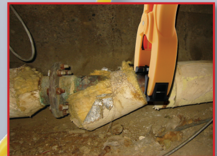
Checking temperature of a failed steam pipe
