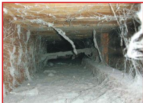
Inspection of hard-to-reach and hard-to-see areas
